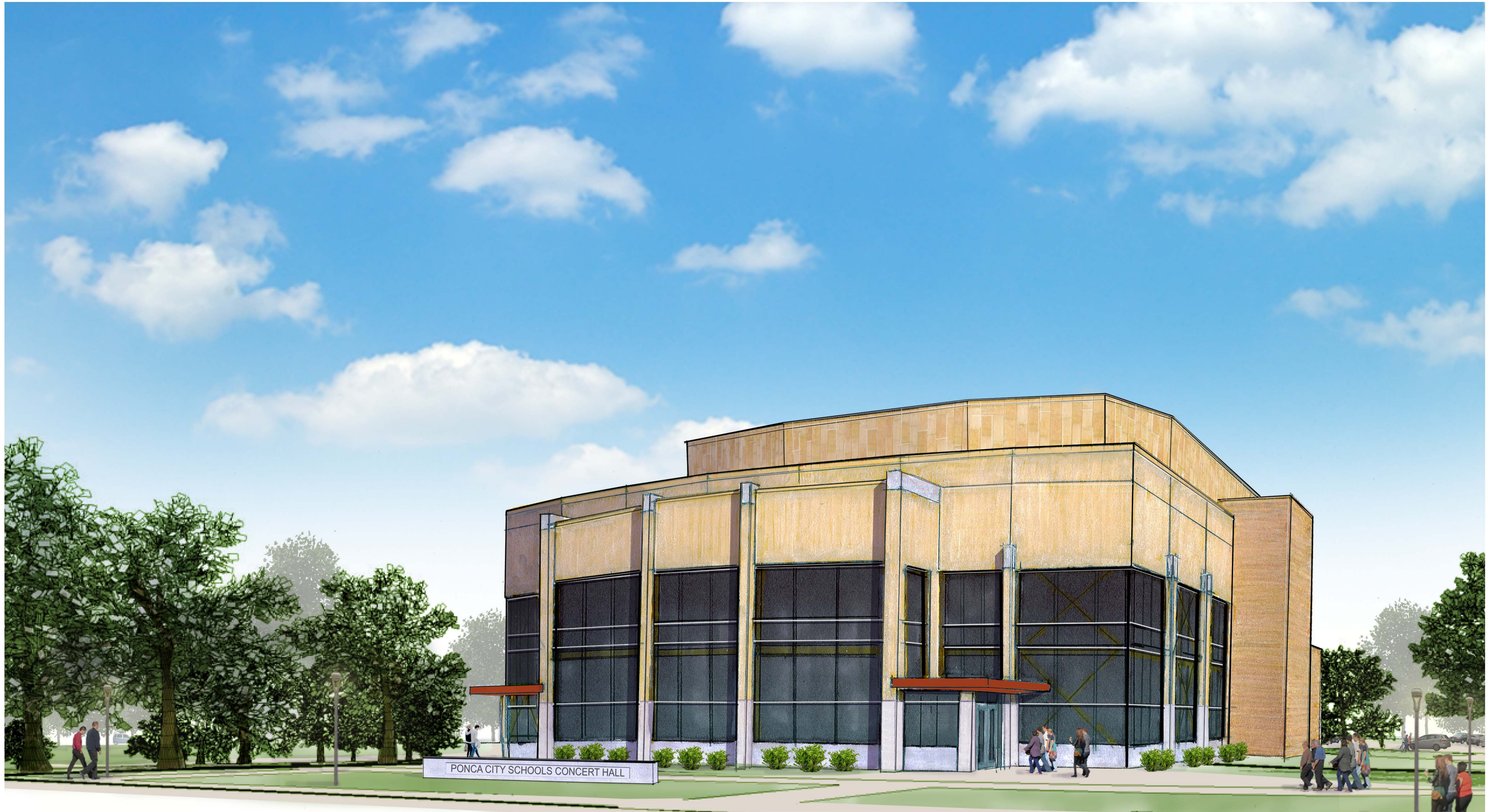
PONCA CITY SCHOOLS CONCERT HALL VIEW FROM THE NORTHWEST
